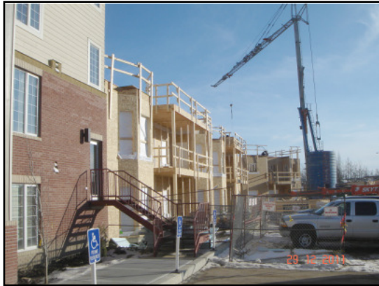
Cranes move sections of roof in Phase II of condo project.
